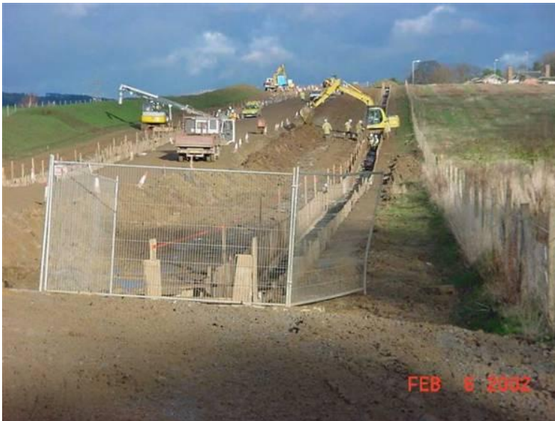
Figure 2-6: Cable Working Swathe for Construction
