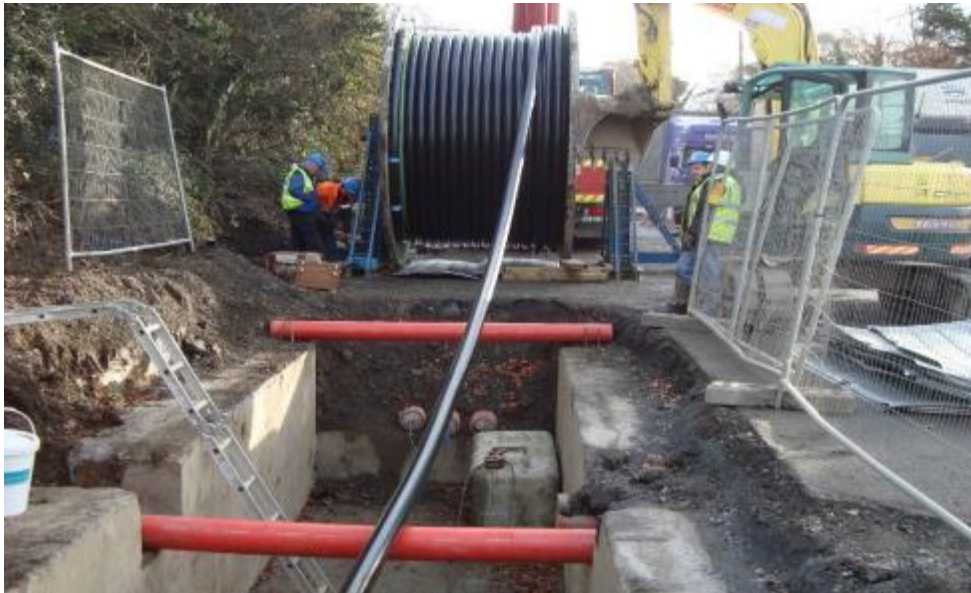
Figure 2-12: HV cable pulling procedure (Typical drum set-up)
