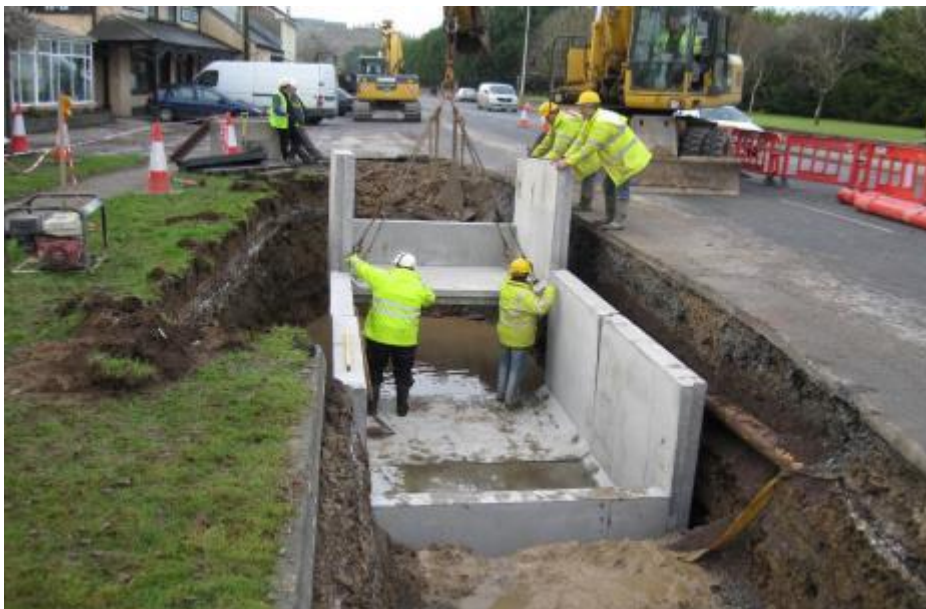
Figure 2-11: Typical joint bay under construction (pre-cast)
