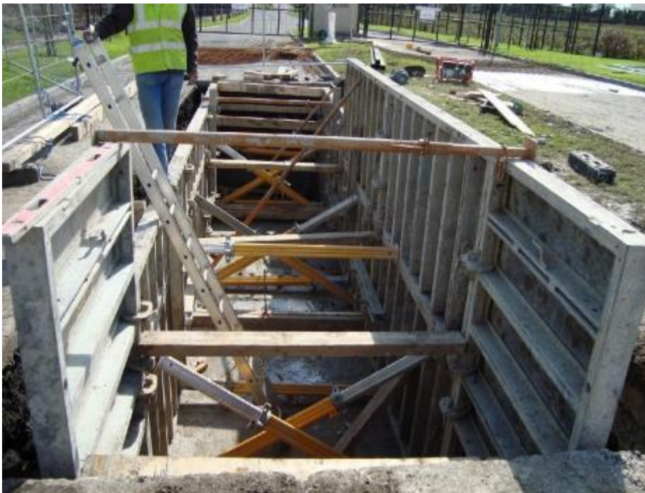
Figure 2-9: Typical joint bay under construction (in-situ)
