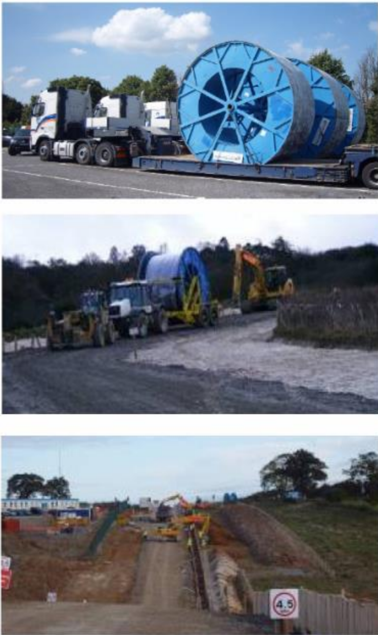
Figure 2-7: Cable Construction Vehicles
