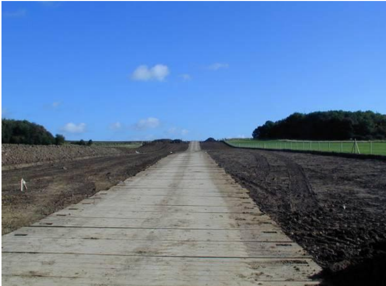
Figure 2-5: Cable Trench Preparation
